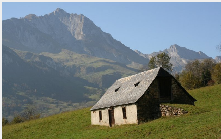
Grange aux Artigaux
