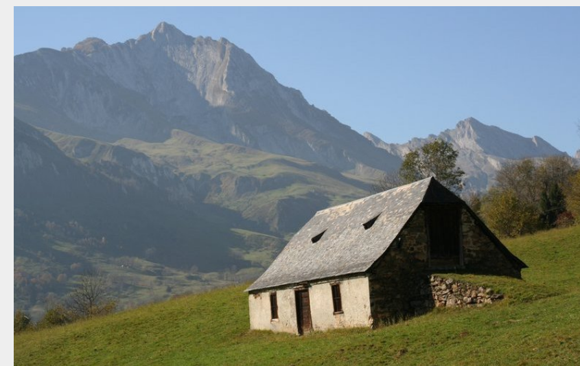
Grange aux Artigaux
