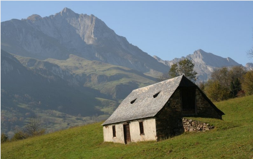
Grange aux Artigaux
